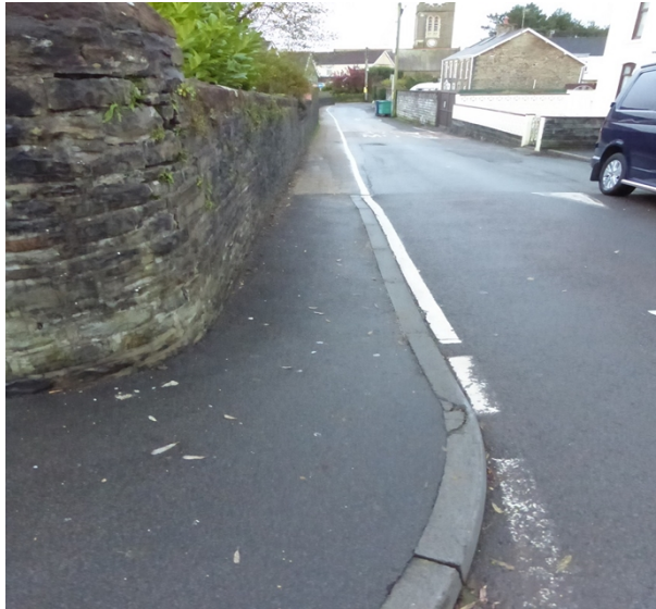
viewed in a southerly direction.
