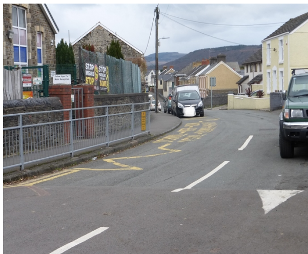
Photograph 1 - Sybil Street showing School Keep Clear Markings and Pedestrian Guardrail
